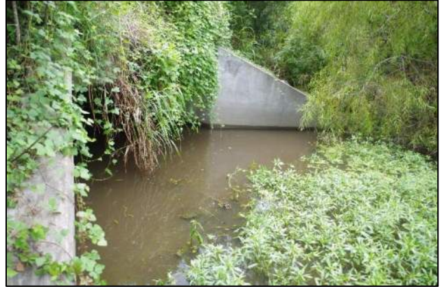
Photo 32. Culvert PC Pkwy Downstream
