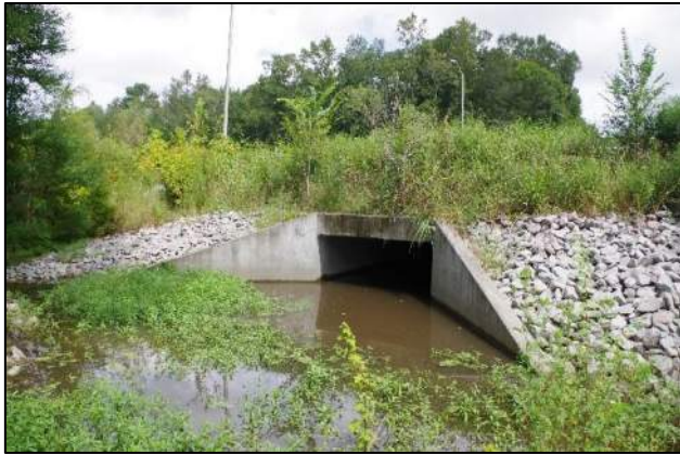
Photo 31. Culvert PC Pkwy Upstream
