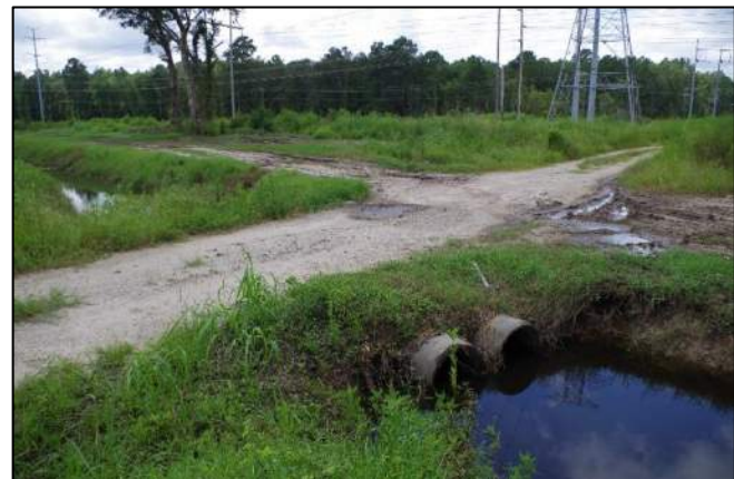
Photo 22. Upstream Utility Road Crossing 8/25/17
