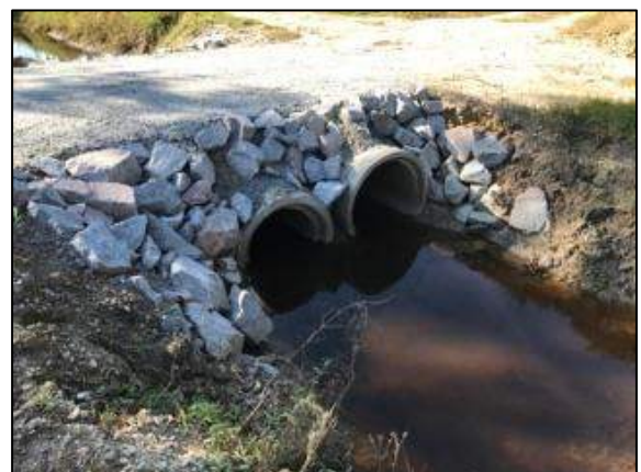
Photo 24. Upstream Utility Road Crossing 11/2017
