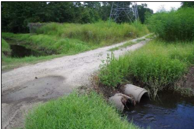
Photo 21. Downstream Utility Road Crossing 8/25/17
