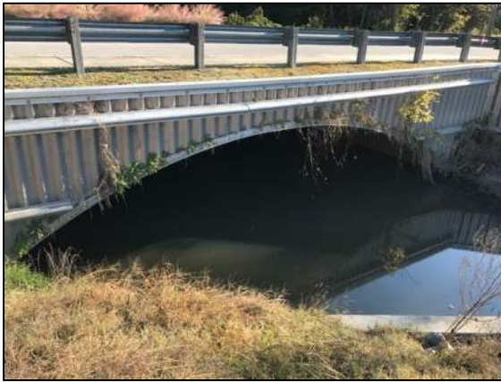
Photo 3. Brookdale Blvd Downstream
