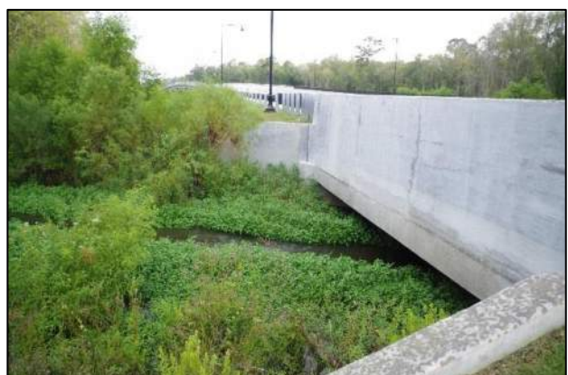
Photo 54. McChune Branch Upstream Weber Blvd
