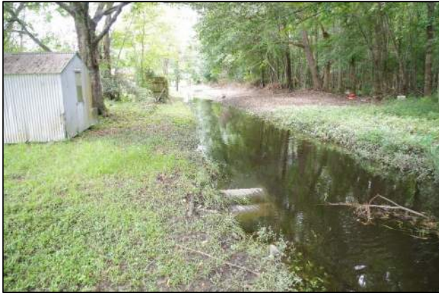
Photo 25. Ditch Full at 7803 Peppercorn Lane 8/25/2017
