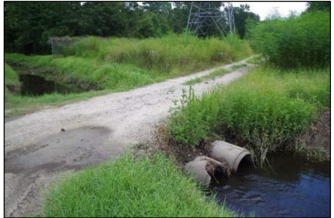
Photo 20. Downstream Utility Road Crossing 8/25/17
