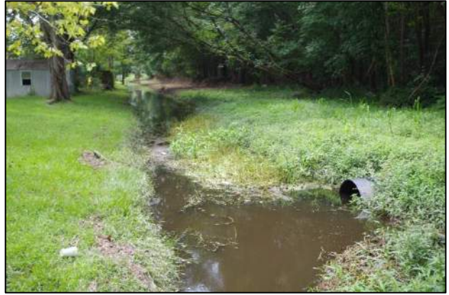
Photo 26. Ditch Full at 7803 Peppercorn Lane
