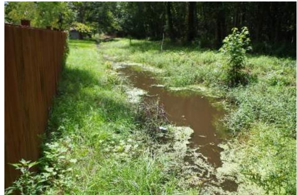
Photo 2-1. Ditch Full at 7809 Peppercorn Lane
