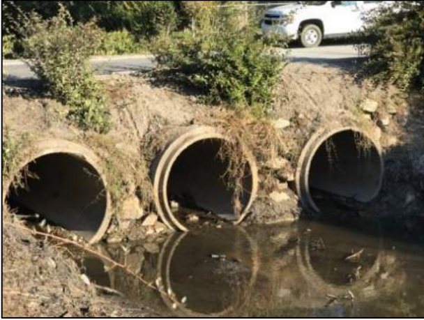
Photo 13. Mountainbrook Road Downstream 11/2017
