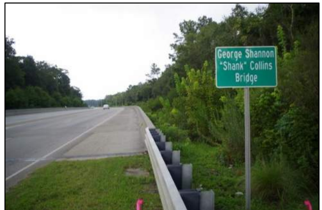
Photo 34. Palmetto Commerce Pkwy Long Bridge
