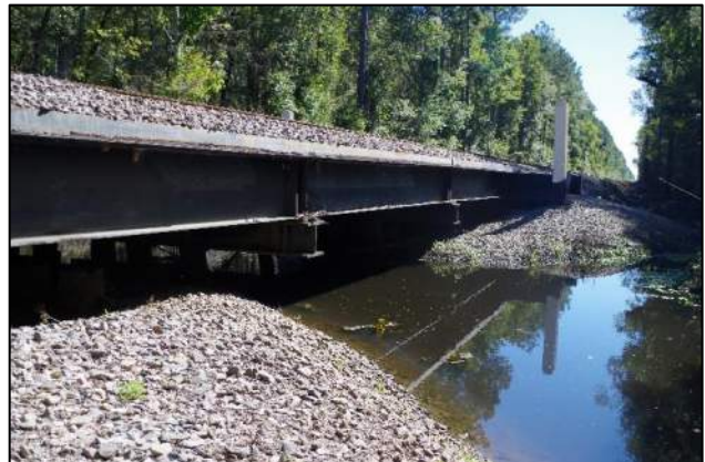
Photo 48. McChune Branch Upstream Railroad Bridge
