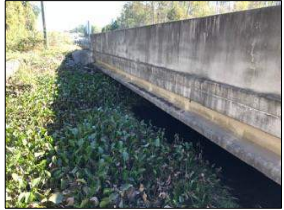
Photo 62. Hwy 78 Bridge Downstream
