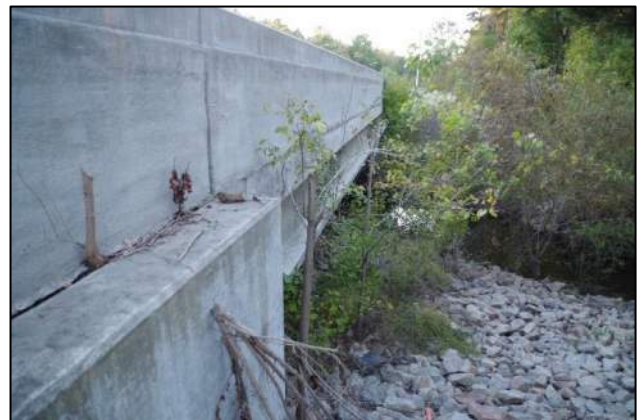
Photo 36. PC Pkwy Bridge over McChune Branch
