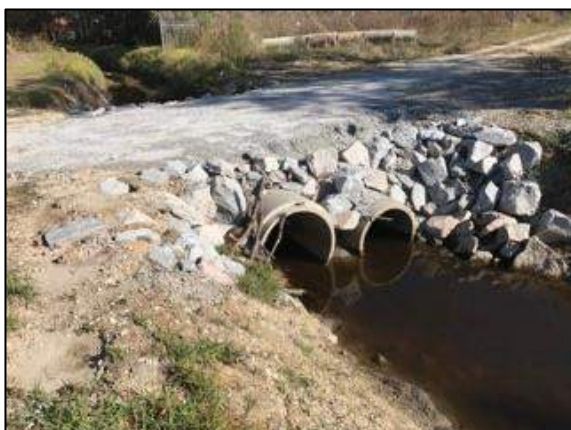
Photo 23. Utility Road Crossing Downstream 11/2017
