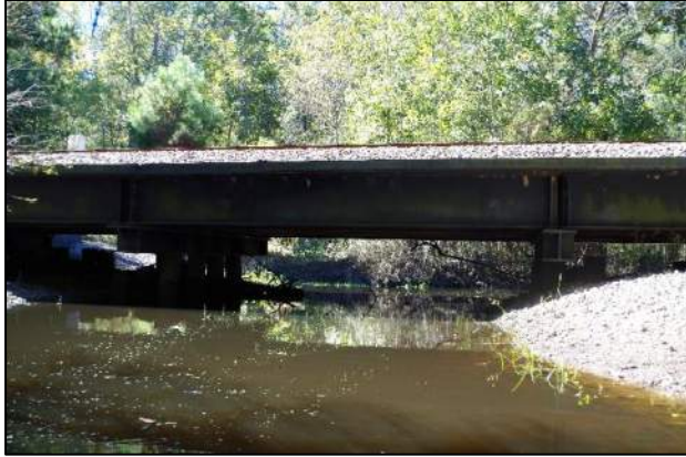
Photo 49. McChune Branch Downstream Railroad Bridge
