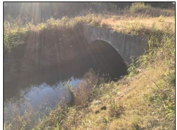
Photo 6. Peppermill Pkwy Upstream
