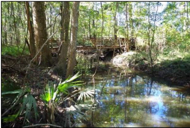
Photo 39. McChune Branch Wood/Metal Bridge
