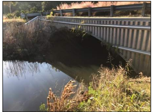
Photo 4. Brookdale Blvd Upstream
