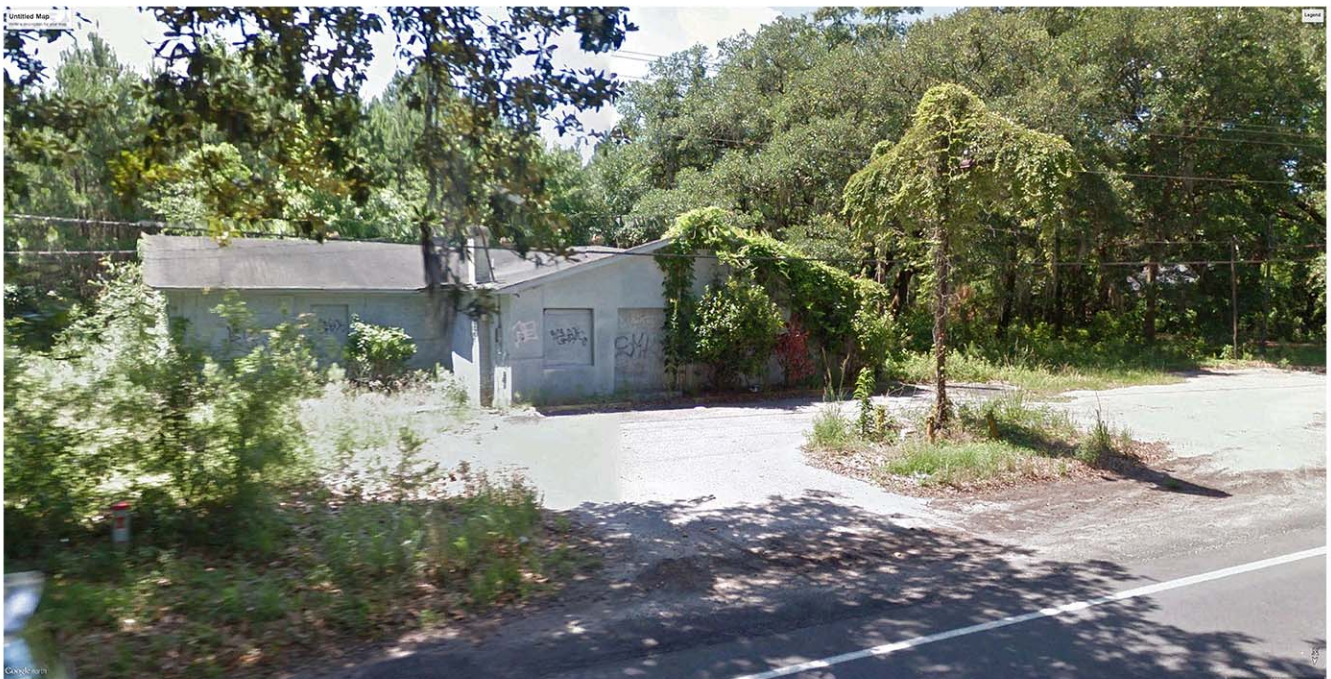
EXISTING ISLAND GROCERY ON PARCEL
