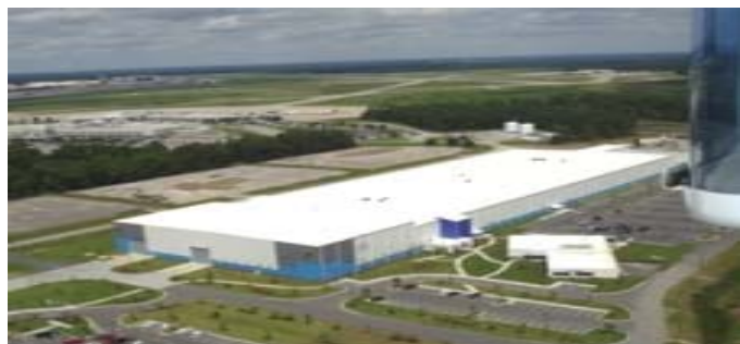
The new Vought Aircraft Fuselage assembly building in North Charleston
