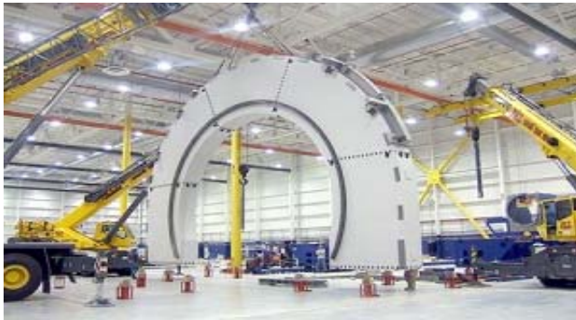
Equipment installation at the Vought Aircraft facility
