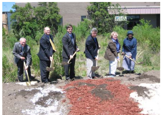
Colleen Condon participates in the groundbreaking ceremony of the port expansion.
