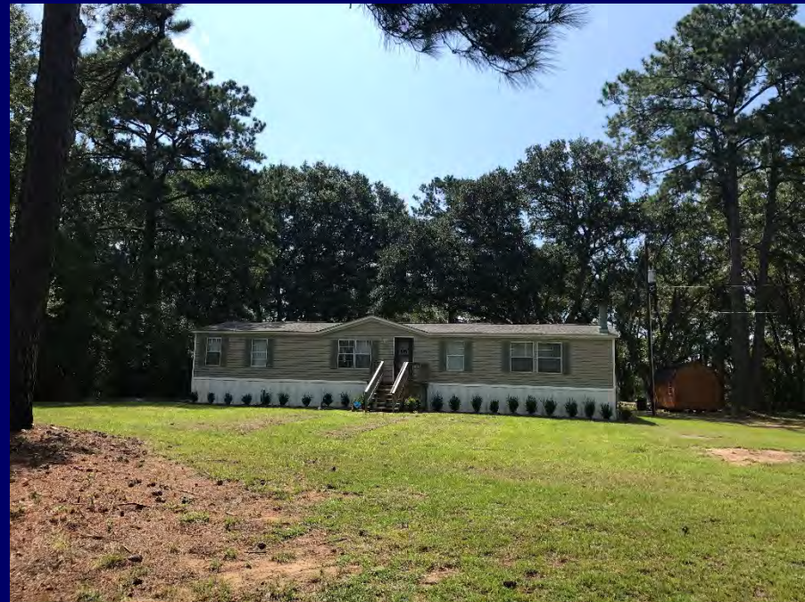
4 – Adjacent Property on Oyster Factory Road
