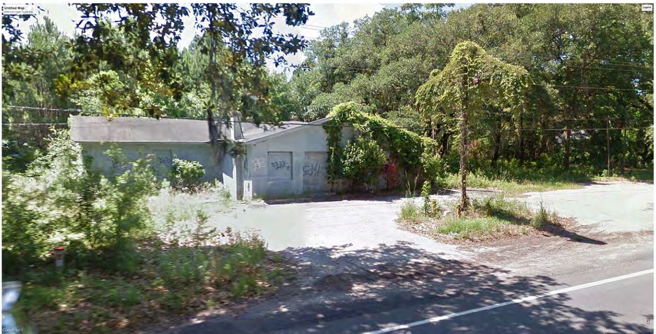
EXISTING ISLAND GROCERY ON PARCEL
