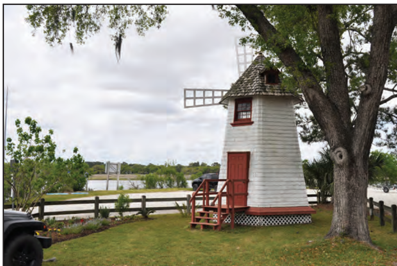
C. Boat Landing, Featuring a Windmill Constructed circa 1939
