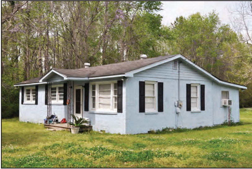
A. Residence Constructed from Concrete Block Resource Number U/19/7339
