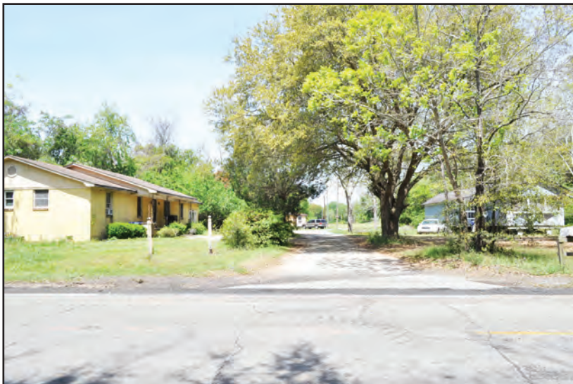
C. Row of Houses on Sol Legare Road
