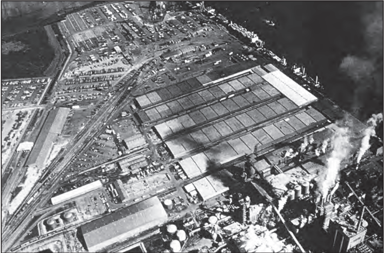
Figure 13. Modernized Port of Charleston Facilities, 1959
