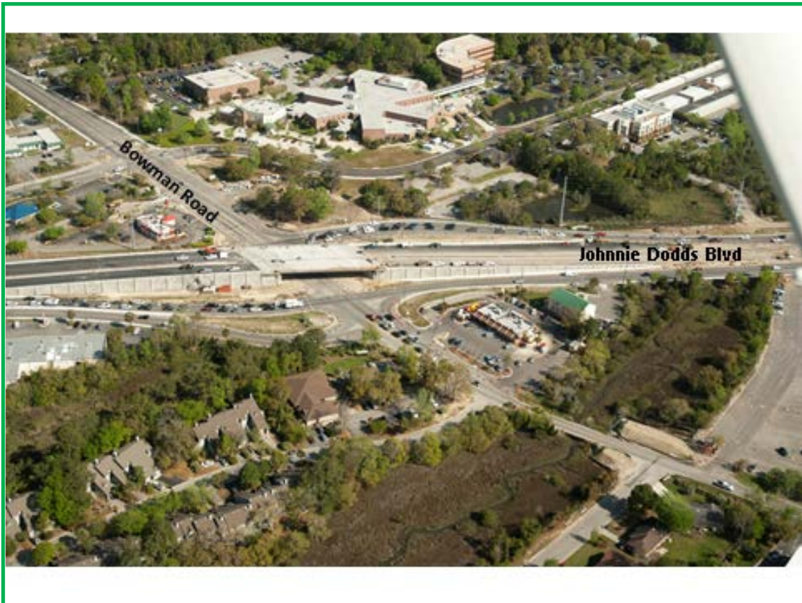
Aerial photo of the new overpass
