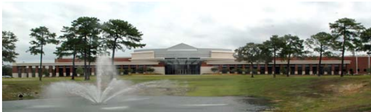
The new Culinary and Hospitality Training Center opened on the Trident Technical College North Charleston Campus in November 2005.
