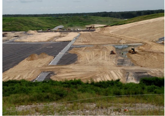
Cell 4 prepared for solid waste
