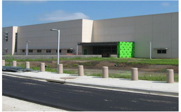
Emergency Services Building on Palmetto Commerce Parkway.
