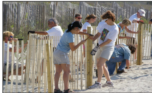
Volunteers install fencing units on Folly Beach, SC
