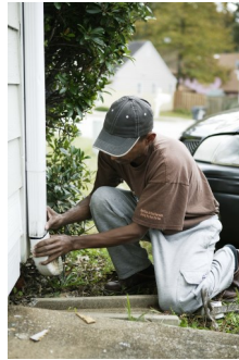
Maintaining your gutters and downspouts. Photo by: David Fine/FEMA
