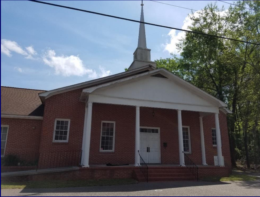
3 – Adjacent Property (Church on Main Rd)
