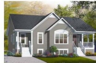
Figure 1 Example of Duplex maintaining residential character
