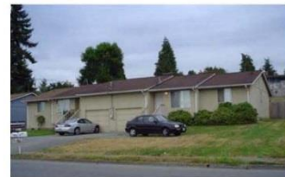
Figure 2 Example of duplex that does not comply with architectural standards
