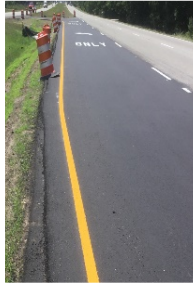
17 South Commerce Center Turn Lane
