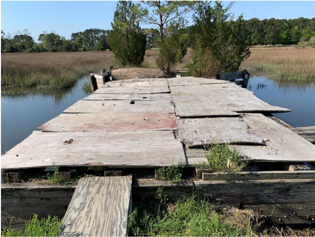
Parker's Island Bridge
