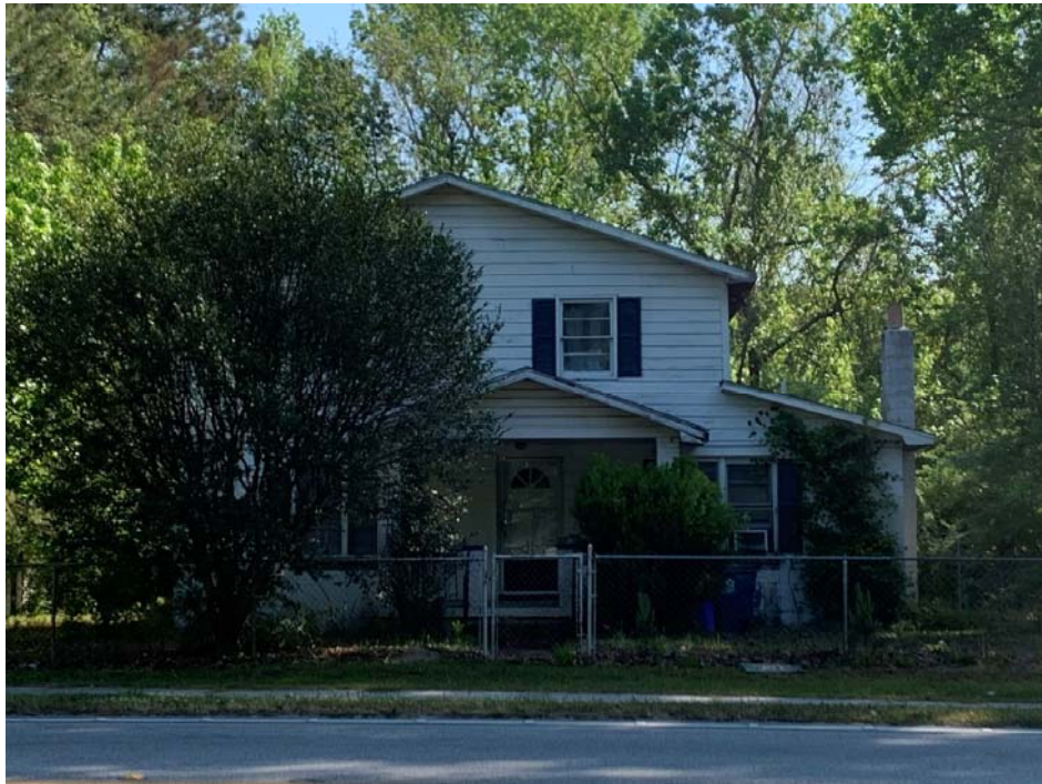
First house with indoor plumbing 1680 Hwy. 41
