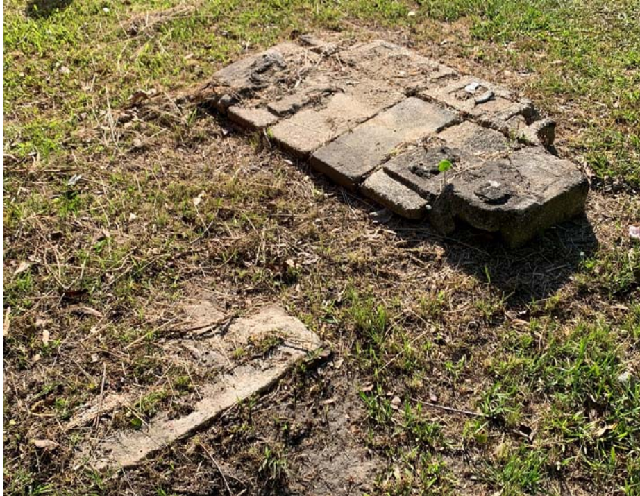
Remnants of Schoolhouse foundation 1749 Hwy. 41
