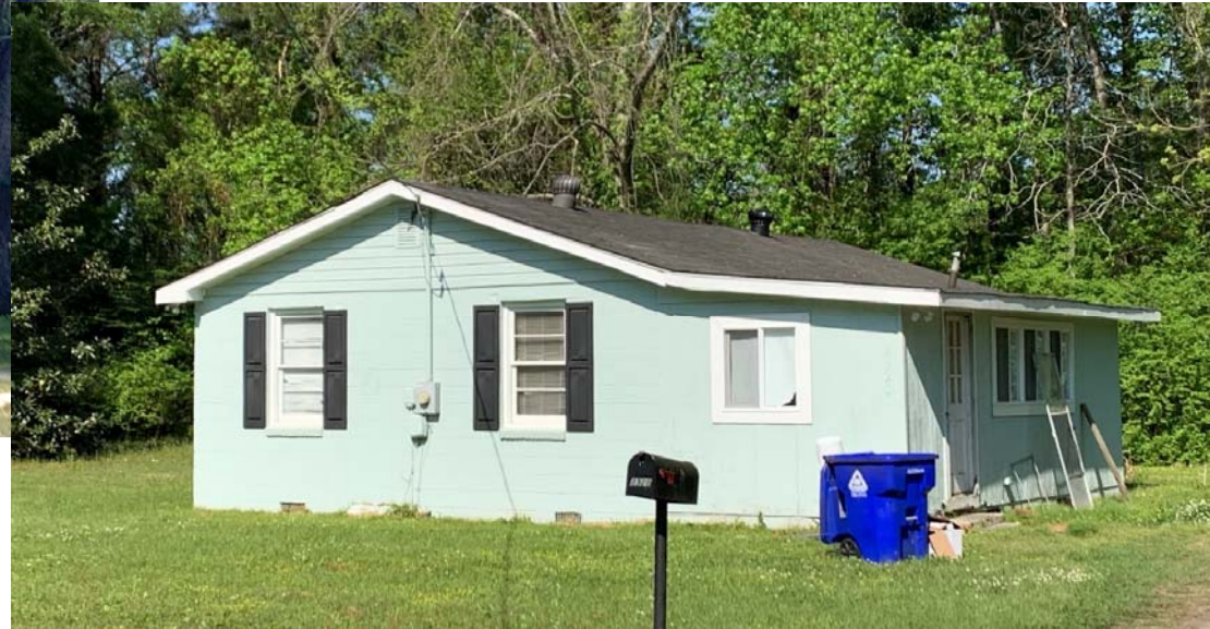
Single Family Home c.1960's (typical) 2920 Bennett Charles Road
