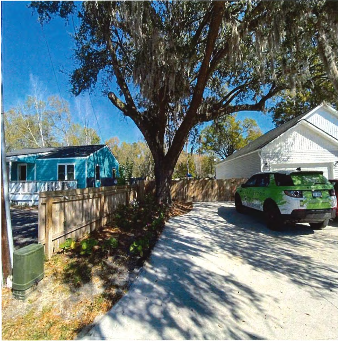
Figure 2: Construction damage caused by excavation of soil to install concrete driveway extension overtop critical root zone (CRZ).
