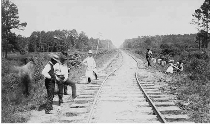
Figure 24. Wilson's photograph after the Charleston earthquake entitled, "Track out of line." This image was taken about 3 miles west of the Rantowles Station, northwest of Johns Island and east of Ravenel.
