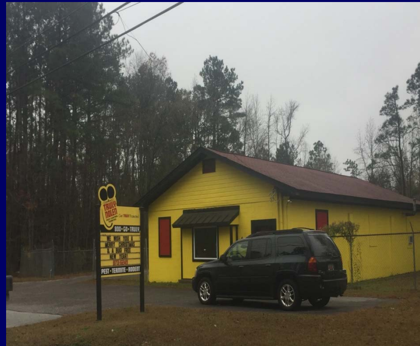
8 – Adjacent Commercial Property
