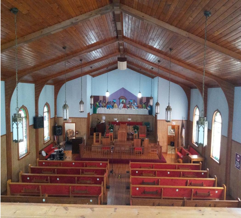
View of the church ceiling with angular wooden beams - note wood panel borders accentuating the blue sheetrock walls
