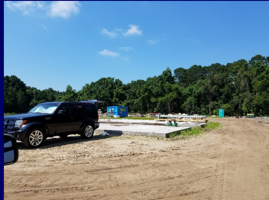
4 – Waste Water Treatment Facility Site
