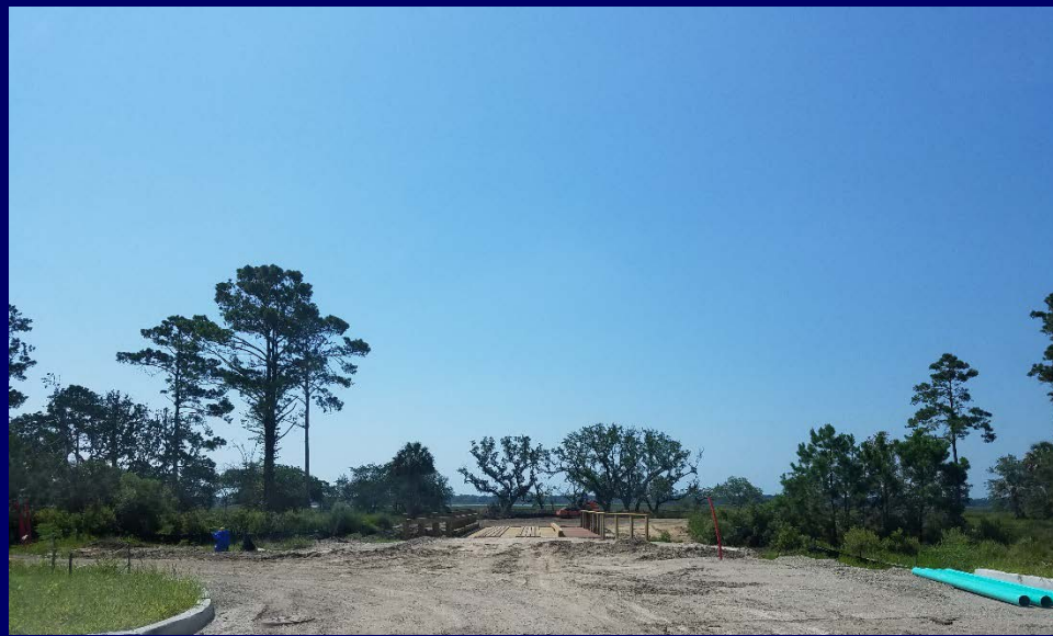
5 – Road on Jack Island & Pedestrian Bridge
