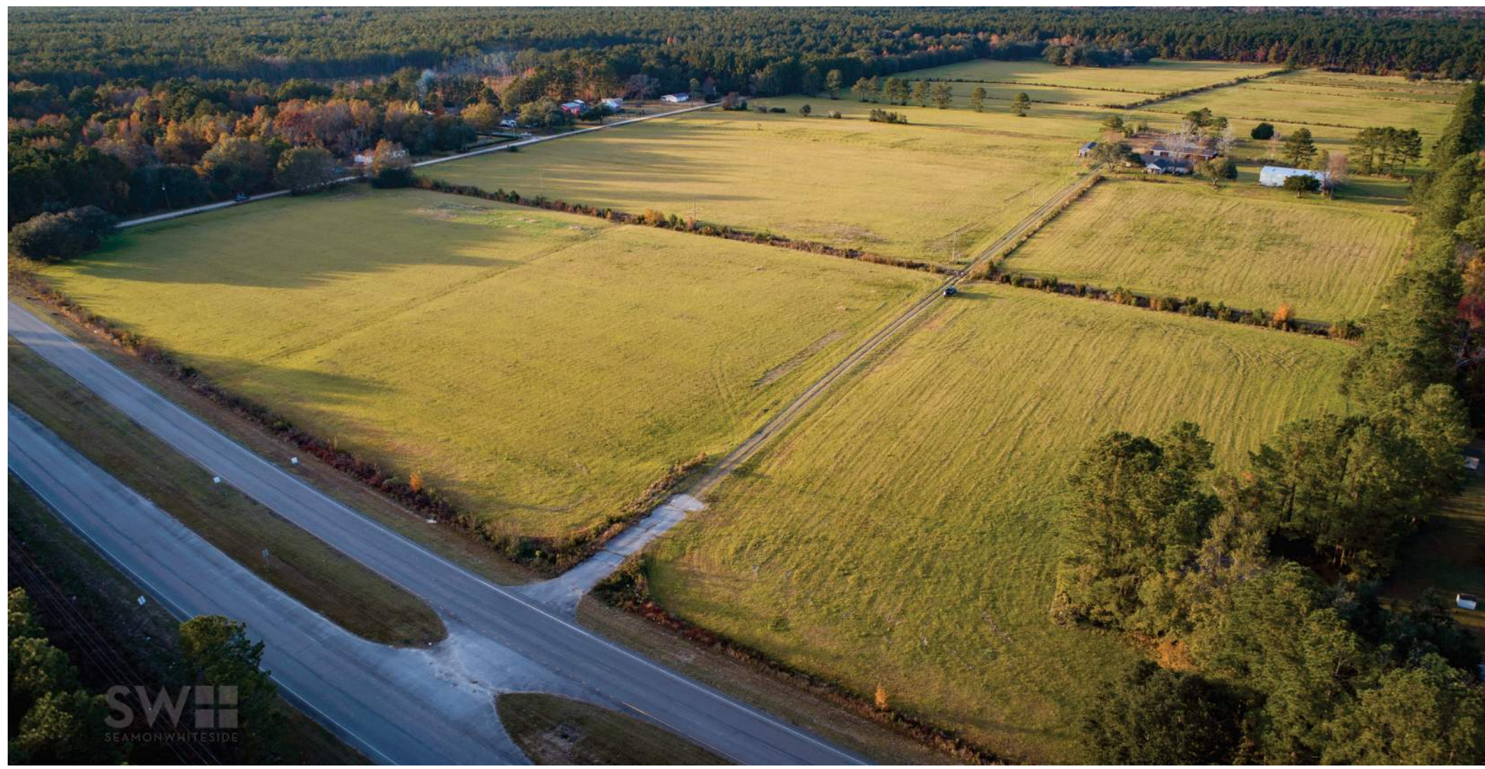
3 VIEW LOOKING NORTHWEST AT SITE FROM HWY. 17
