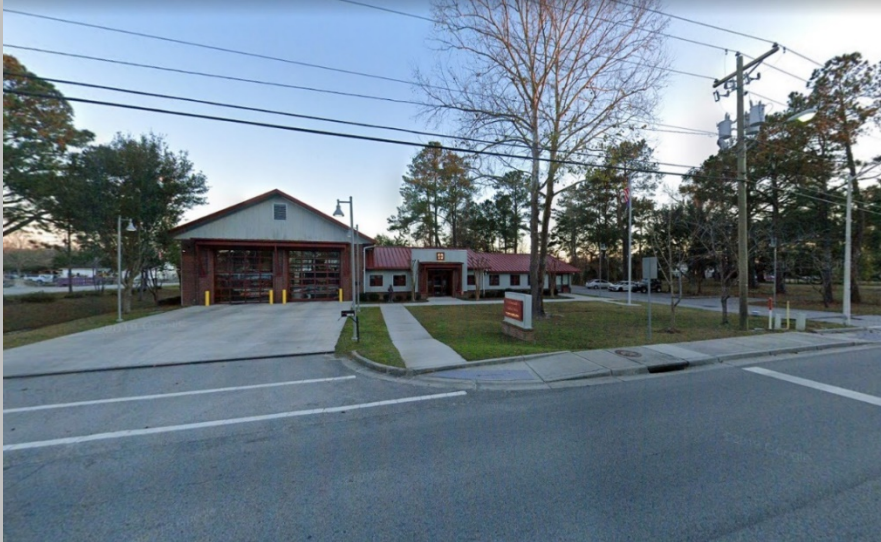
Fire Station District 19 TMS 356-00-00-034
