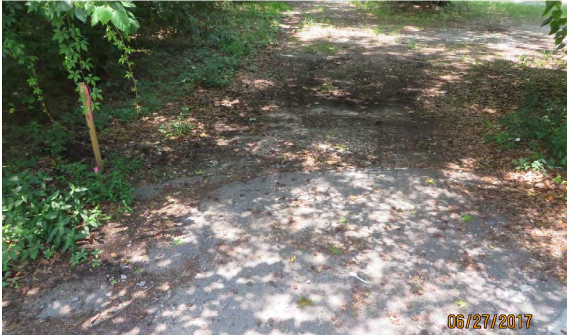
F: Westerly View of Southern Gravel Drive
