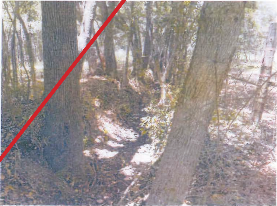
Figure 14 - View looking northwest at existing ditch
