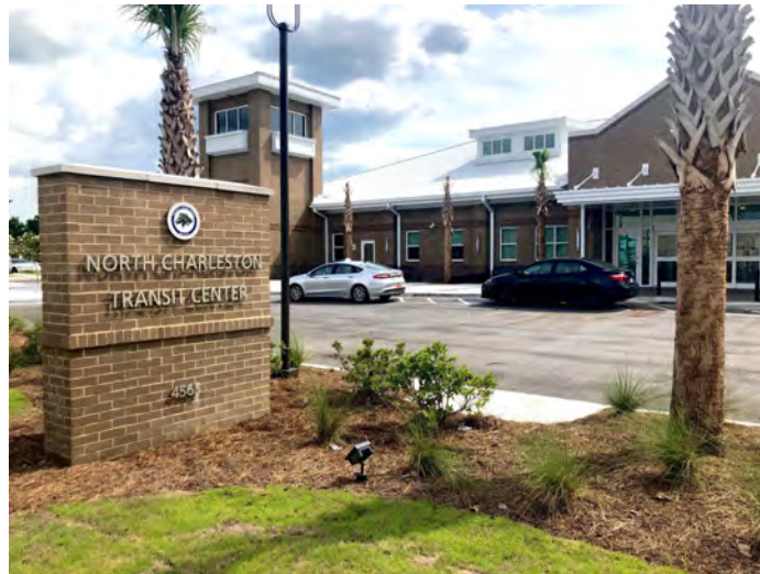
North Charleston Transit Center (Source: www.davisfloyd.com)
