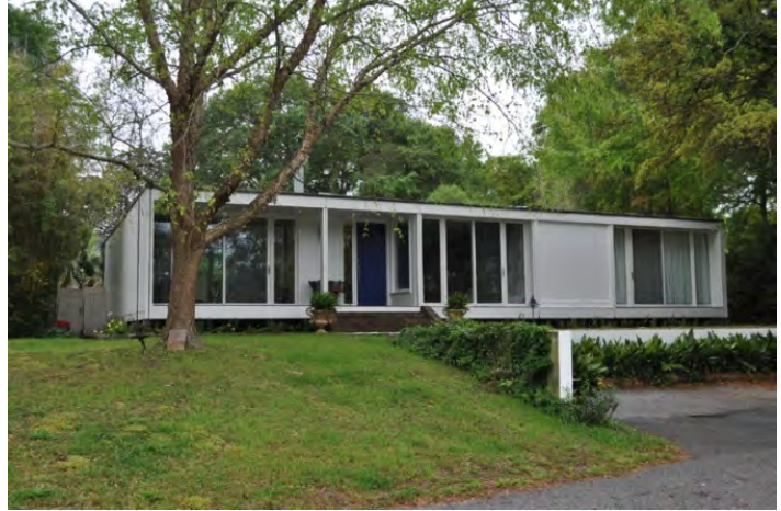
Elliott Constantine House in Riverland Terrace
