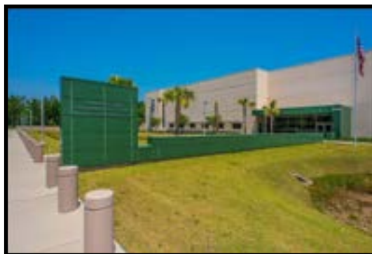
Charleston County Consolidated 9-1-1 Center and Emergency Operations Center
