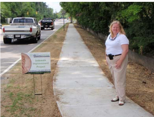
County Councilmember, Colleen Condon, checks out the completed Charlestowne Drive Sidewalk Project. Residents living in Charlestowne Estates II and the Lenevar subdivisions are now connected by 2,100 feet of sidewalk that will also tie them to Charles Towne Landing State Park.
