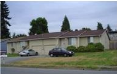
Figure 2 Example of duplex that does not comply with architectural standards
